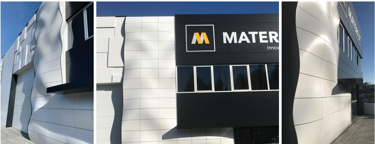
A new option to create, saving time and reducing resources and environmental impact - for exterior and interior cladding solutions with complex geometries and structures, curves and irregular shapes (photos: exterior cladding project for Materfut® building, Portugal).
